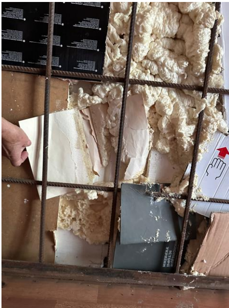
Russian troops used Ukrainian library books as construction material to plaster walls in the destroyed Village Culture Club, Village of Peremoha, Kyiv Region. Photo Khanenko-Friesen.
